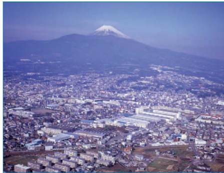
The Toshiba Machine Numazu Plant in Japan
